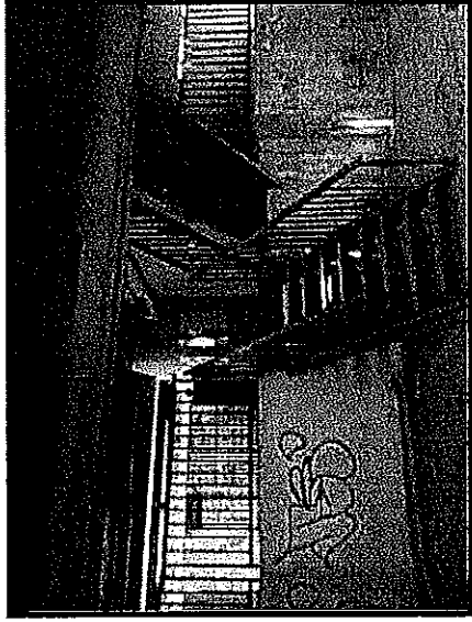
From basement to first floor
