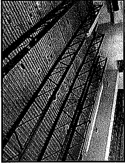
Steel truss roof and panels
